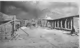
THE ROMAN CATHOLIC church of Sabana, is being planned by the construction of the new quarters of the Christian Brothers' community. Lago donated Fls. 33,000. To be completed the latter part next year, it will house 15 to 18 Frere.
